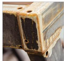
**External venting in hollow section frames.** The photo shows a RHS fabrication. The hole size is adequate, however the holes should be nearer the corner of each member.
